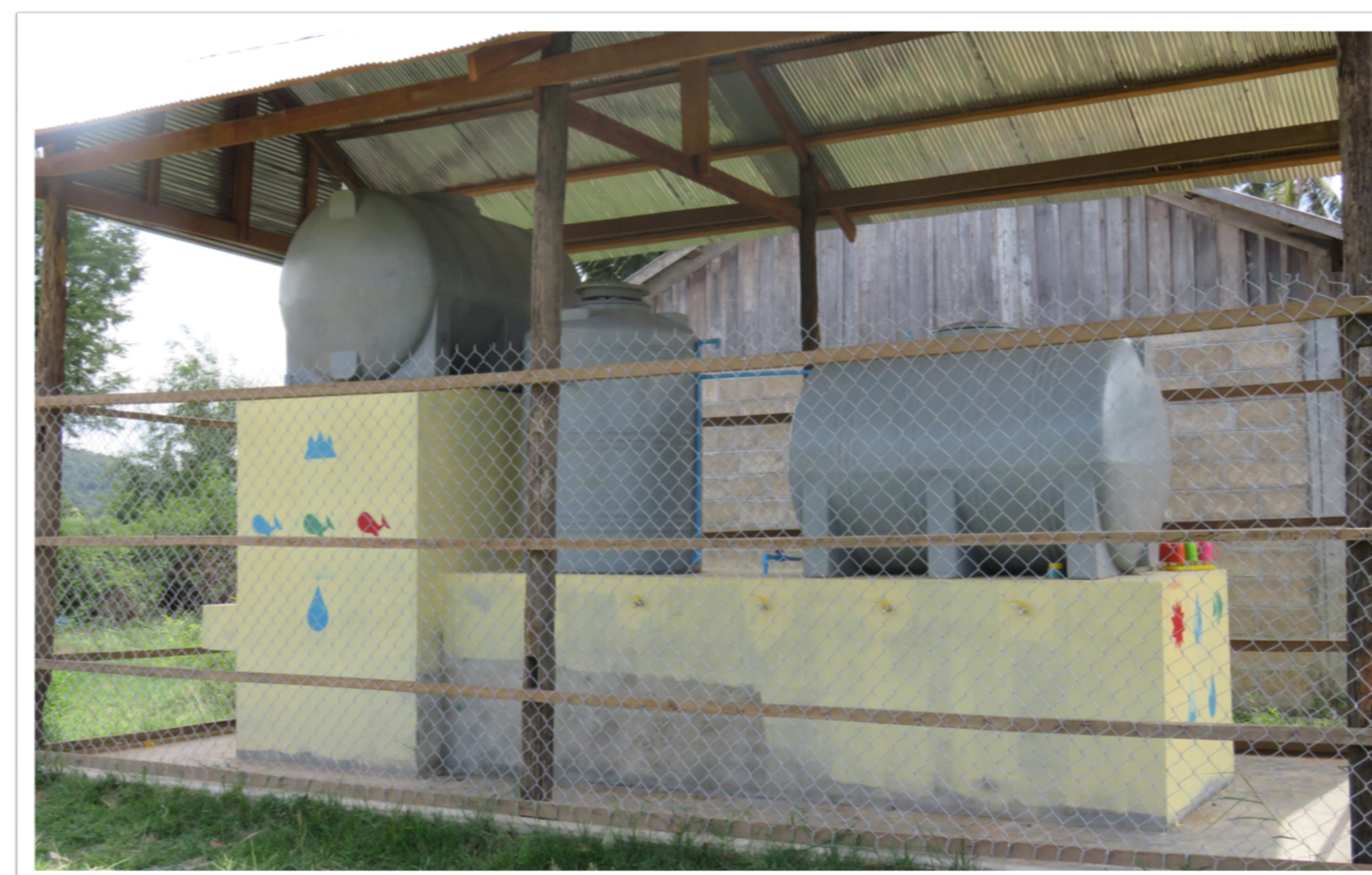
Figure 2: Typical slow sand filter installation
